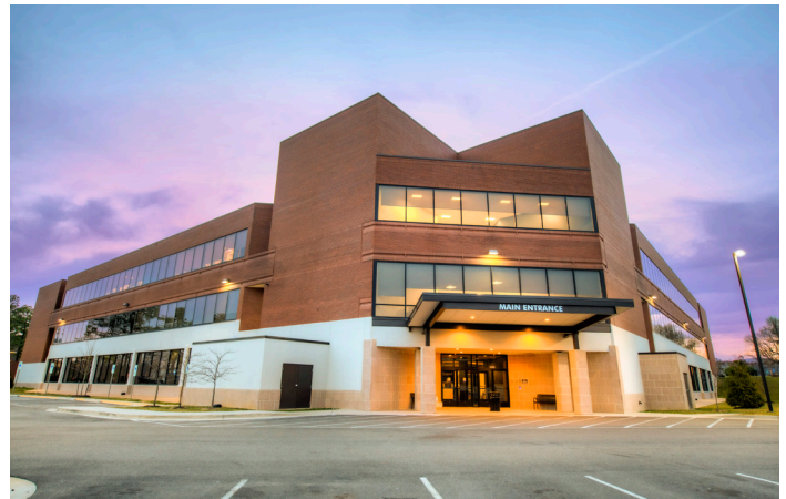
Brookfield Commons MOB, Richmond, VA One Building | SF 90,000
